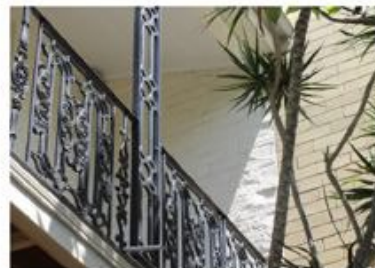
Original detailing restored and repainted
