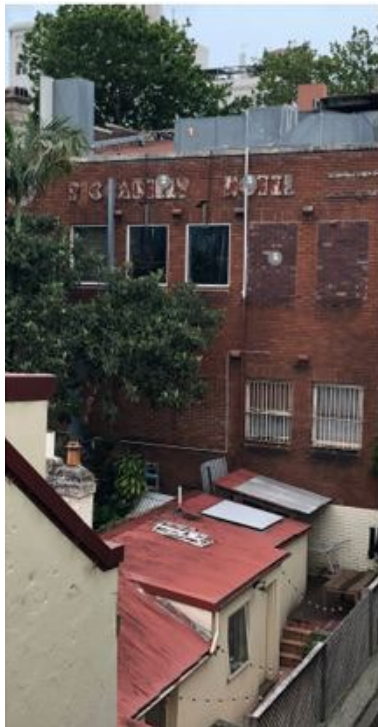
Current image of the west facing Piccadilly facade, showing signage, bricked in windows and roof plant
